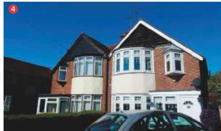
Existing residential buildings located on the site
