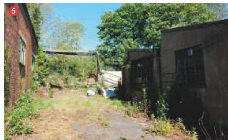
Site sloping up to vegetation buffer and train line
