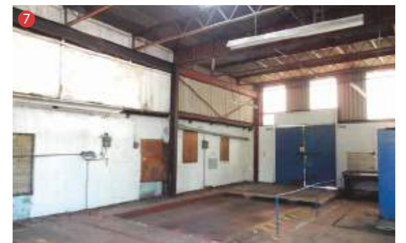
Inside one of the industrial buildings
