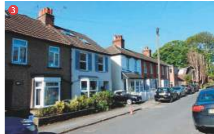
Houses along Bower Vale
