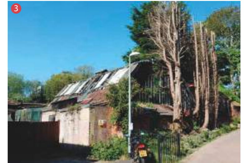
Existing laundry building facing onto Bower Vale
